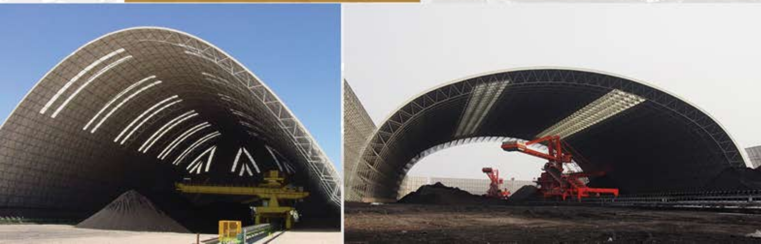
Coal Handling Sheds
