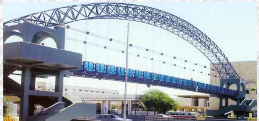
Pedestrian Suspended Arch Bridge
