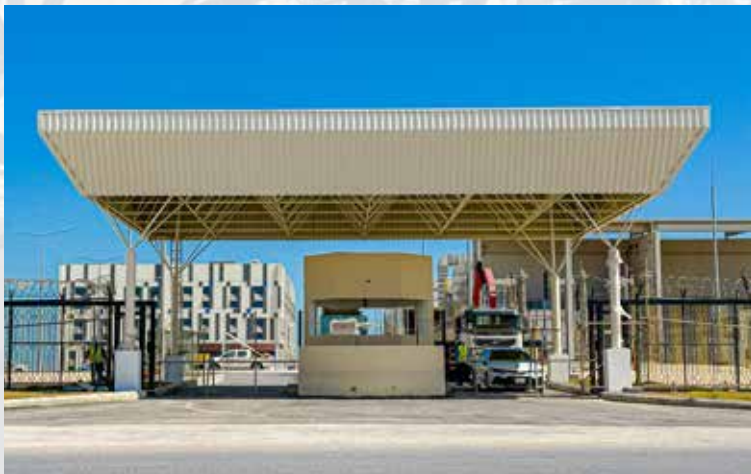
SWCC Security Gate Sunshade, Jubail
