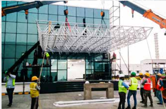
2 . BLOCK ASSEMBLY METHOD
